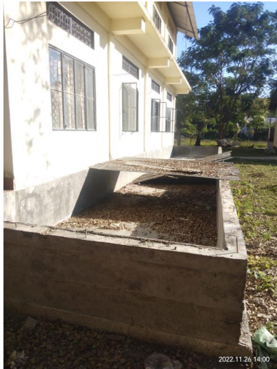
Figure 11: Rain water Harvesting System (Under construction stage)
