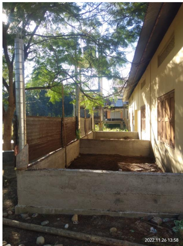
Figure 10: Vermi-Compost Unit (Under construction stage)
